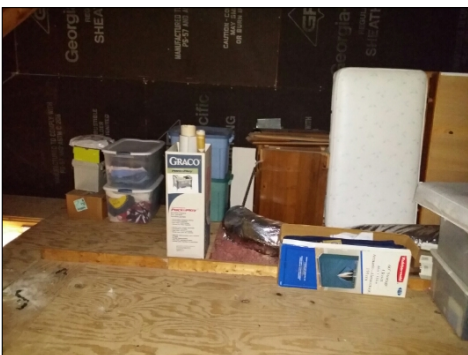
Storage limits visual inspection
