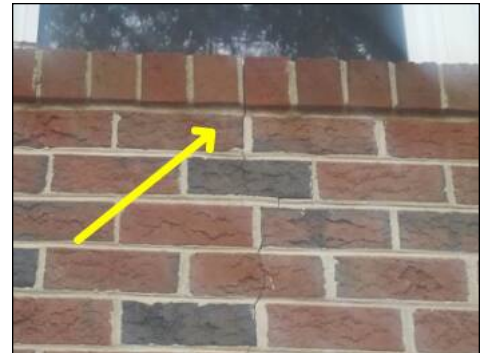
Cracked brickwork
