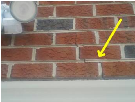
Cracked brickwork
