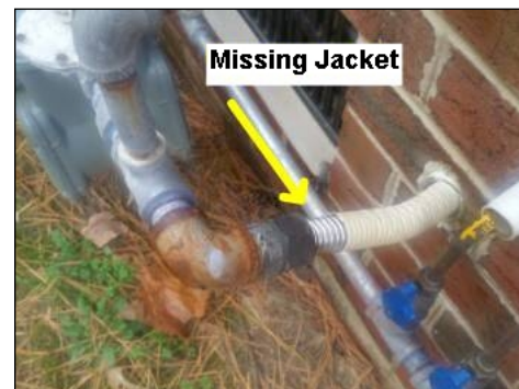
No additional bonding for CSST
