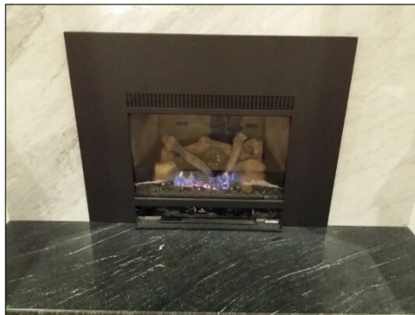
Pre-fab gas fireplace
