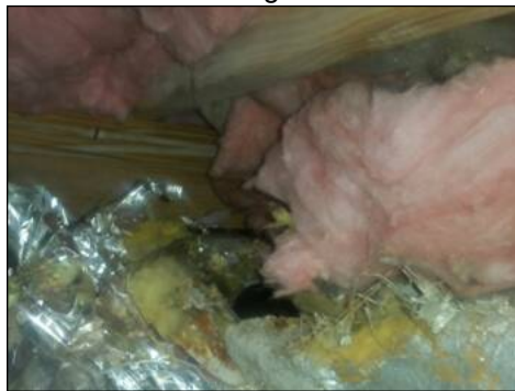
Disconnected ductwork
