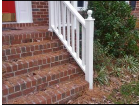
Loose handrail
