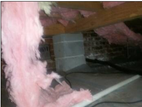
Falling insulation
