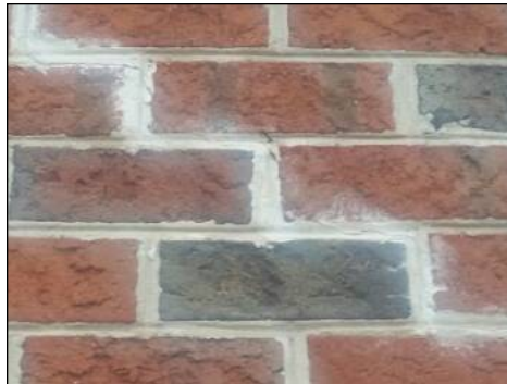
Cracked repairs
