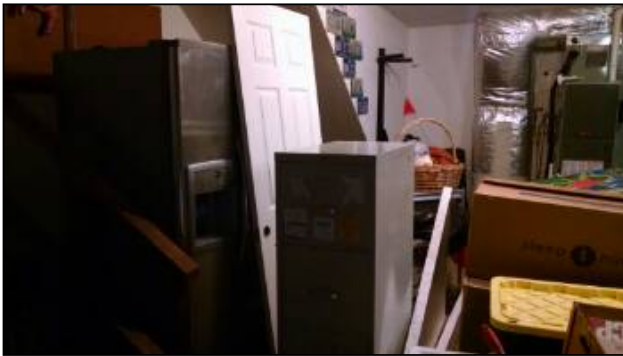
Storage limits visual inspection
